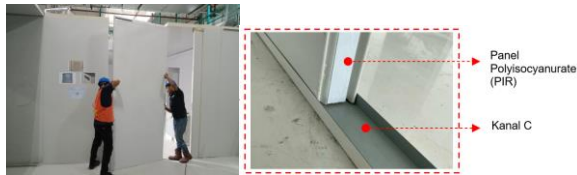
(c) Pemasangan Panel Polyisocyanurate
